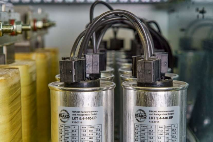
Photo 1. FRAKO power capacitors are 'Made in Germany' and incorporate a fourfold safety system for maximum operational reliability.
